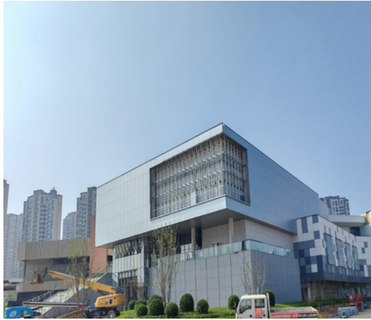
Fabrication of steel structure
