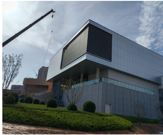
Install the LED display cabinet
